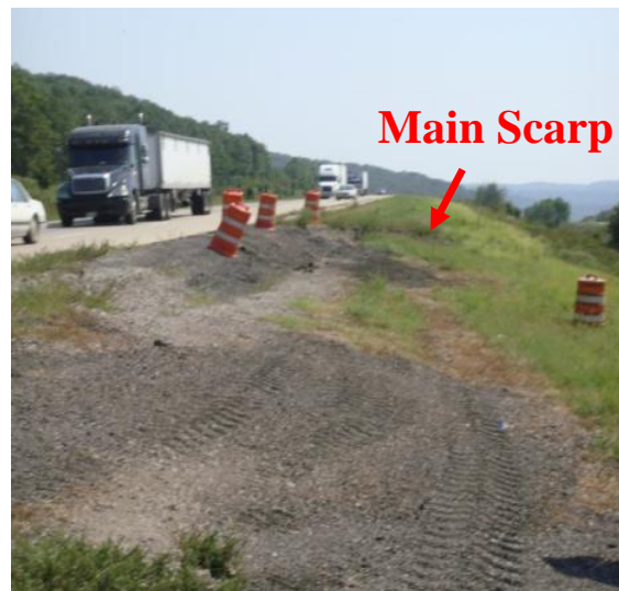
Figure 3.7. Traffic passing next to the main scarp in calibration site near Chester, Arkansas.
