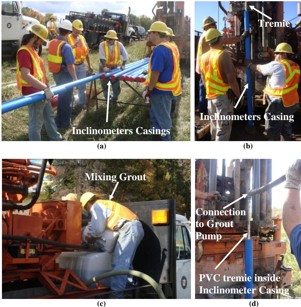
Figure 4.36. a) Sections of inclinometer casing, b) installation of inclinometer casing, c) preparing grout mix, and d) grout connection between tremie and grout pump.
